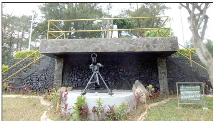
Concrete floor extension of the wreath laying area at Departed Alumni Memorial
