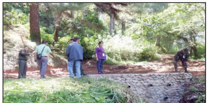
Construction of soil erosion control structure at Eco-Trail Area
