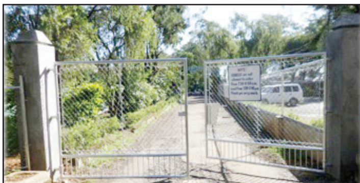
Perimeter fence and steel gate at FDP Elementary School
